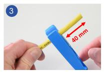
Using an appropriate stripping tool, remove approximately 40 mm of the cable jacket from the data cable.
