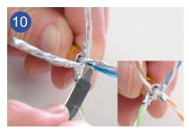
Cut all pair-shield tapes with a side cutter down to 5 mm.
