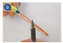
Cut the pairs oblique with a side cutter.
