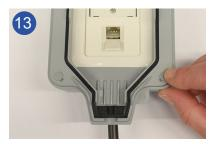
Mount the cover with the four long self-tapping screws and seal the openings with the four grey plastic plugs.
