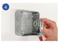
Tighten the nut of the cable gland firmly with channellock plier.
