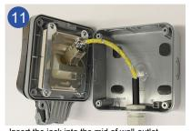
Insert the jack into the mid of wall-outlet until the lower mounting spring clicks into place in the metal frame.
